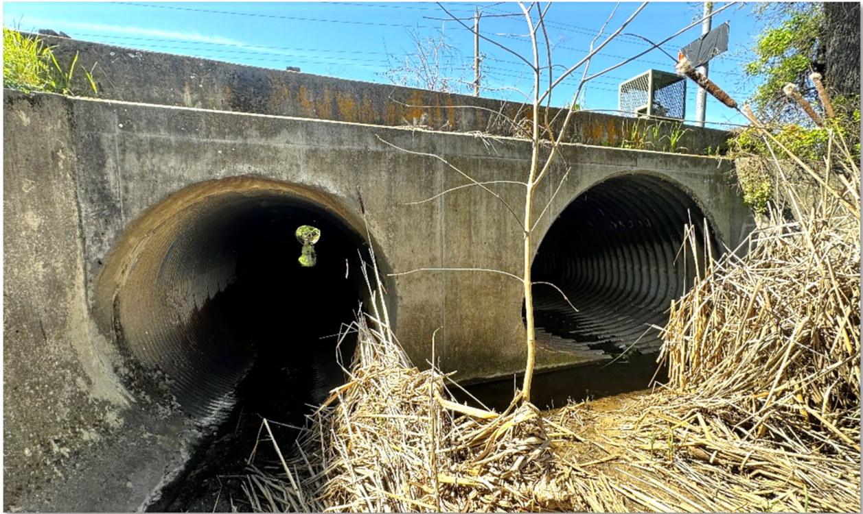
Figure 16. Sunrise Ave Culvert Crossing (looking downstream) at Cirby Creek (R&F, March 2024).
