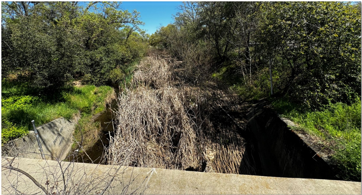
Figure 17. Sunrise Ave Culvert Crossing (looking upstream) at Cirby Creek (R&F, March 2024).
